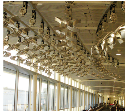
The implementation of the artwork at San José International Airport makes use of the convenient modular nature of SmartMotor™
